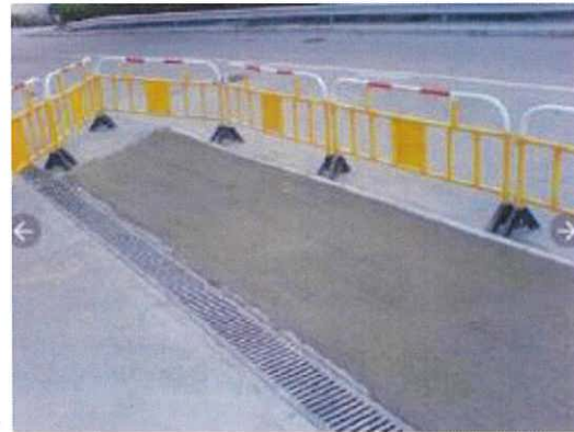
(f) Spare PVC ducts marked on the footway thus C↑D
