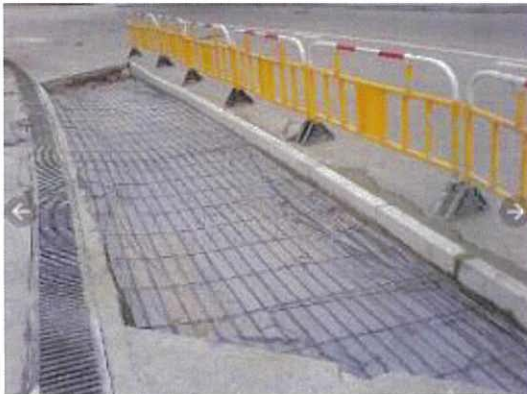
(e) Concrete paving
